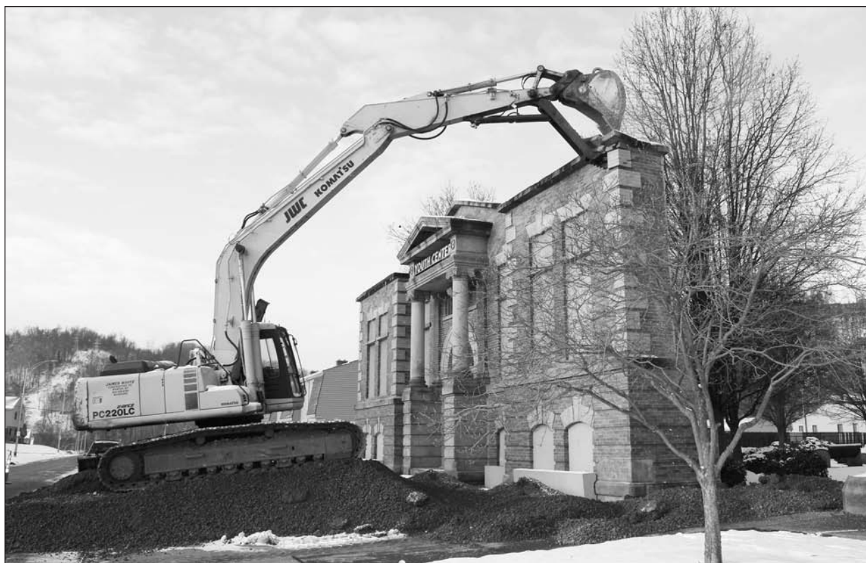
Work continues by James White Construction Co., Weirton, West Virginia, to set the stage for a renovated, restored and renewed Holy Name Cathedral, Diocese of Steubenville Bishop Jeffrey M. Monforton told the diocesan Presbyteral Council Feb. 11 in St. Clairsville. The facade of the former Youth Center that stood next to the cathedral rectory on South Fifth Street, Steubenville, is being removed to permit realignment of streets to create a pedestrian-friendly walkway. (Photo by DeFrancis)
